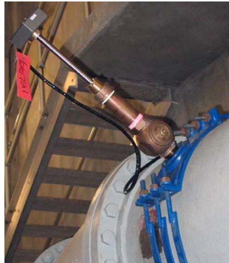
Hot Tap sensor installed in 30" ductile iron pipe
