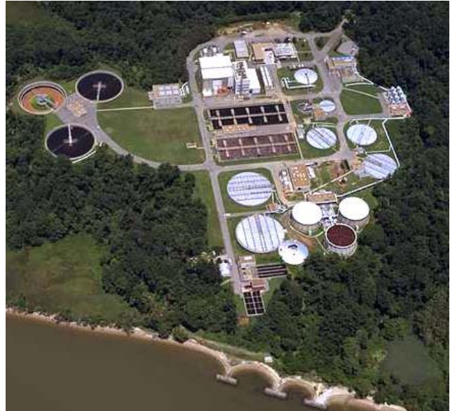
Photo of Williamsburg Treatment Facility courtesy of HRSD
