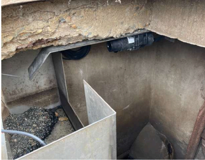
Installation with angle rebate mounting kit
