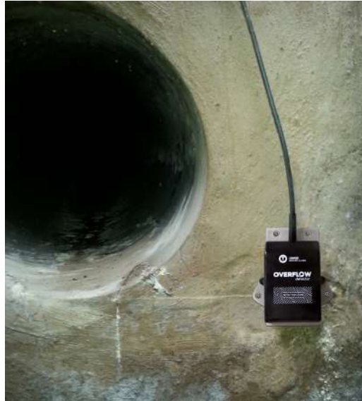
Installation in storm drain
