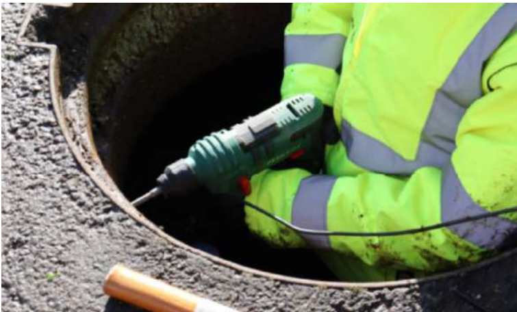
Drill hole in manhole
