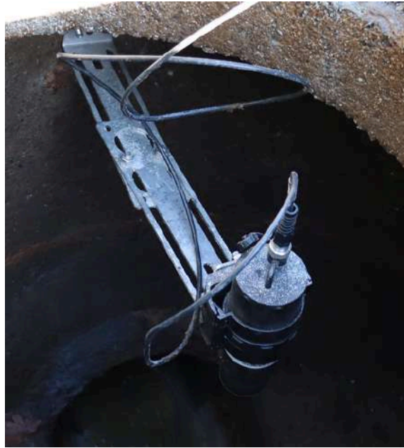
Example of installation with two mounting plates
